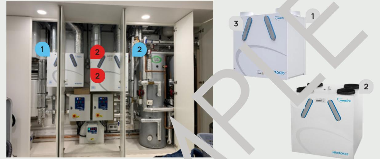
It is required to clean and eventually replace the **Filters 3** on the front of the Unit every **12-18 months**. The heat exchanger and motor should also be checked. To order new filters scan the QR code on the front of the Unit.
