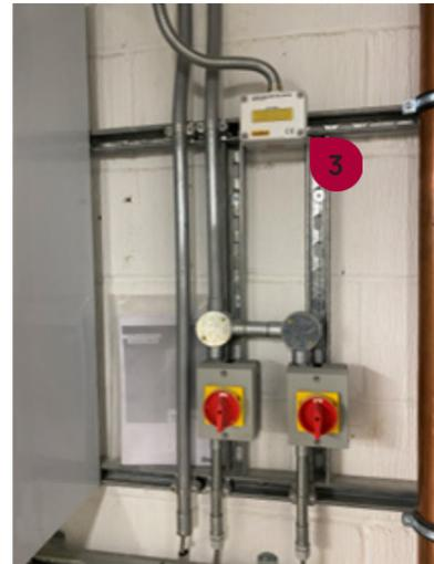
The Boilers should now start and the digital temperature gauge should increase to approximately **60°C** to **65°C** (unless there is an external problem).
